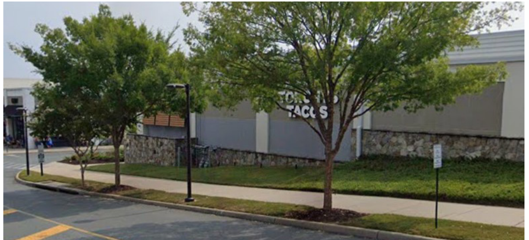
VIEW OF TORCHY'S RETAINING WALL AT HYDRAULIC RD AND SWANSON DR
