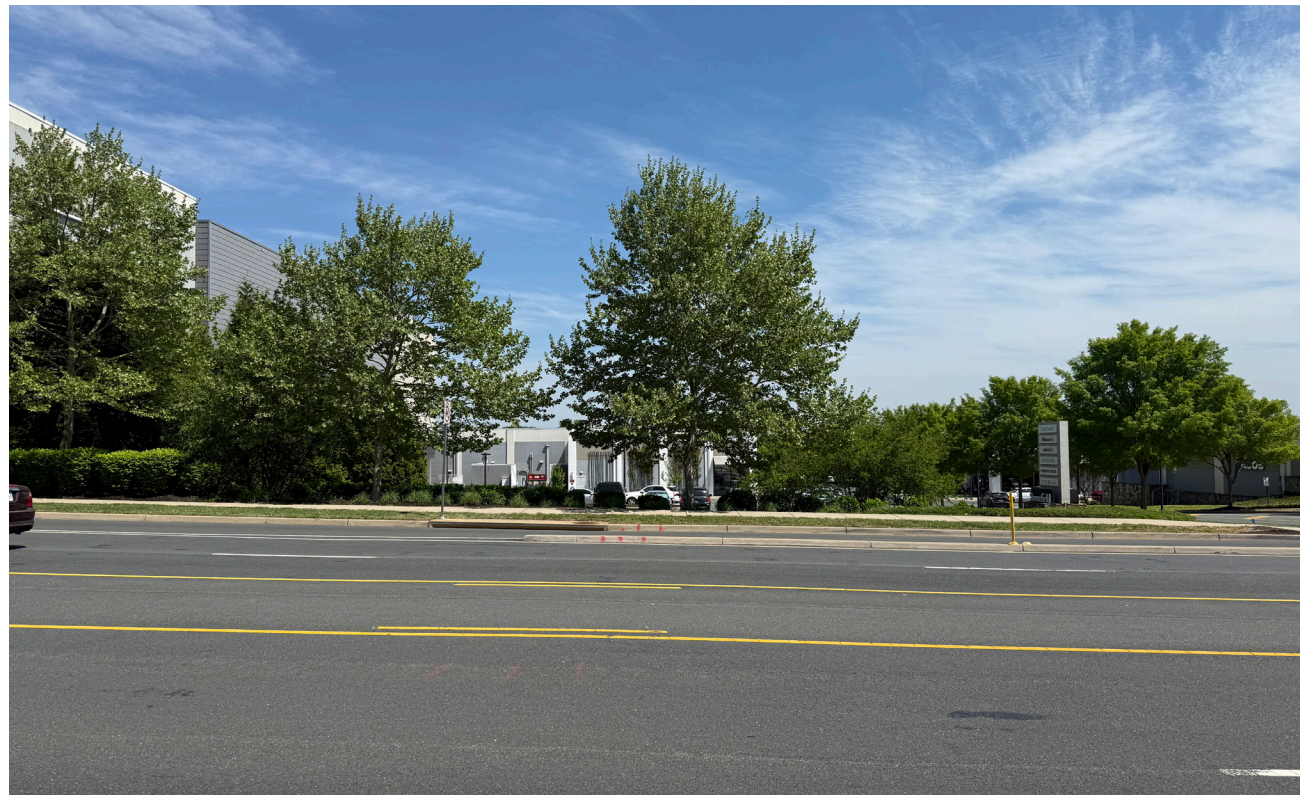
VIEW OF SITE FROM ACROSS HYDRAULIC RD
